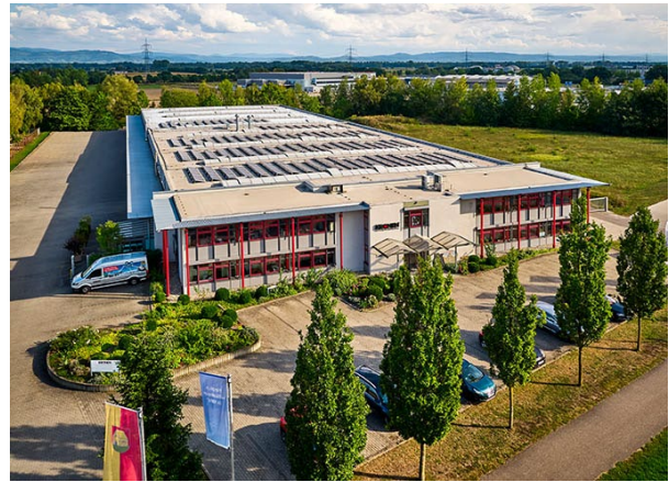
The company building of KRONEN GmbH in Kehl: the machines and processing lines manufactured here are delivered to customers all over the globe.
